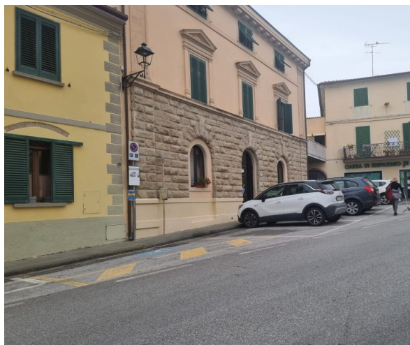
Figures 4 Reserved stall in via del Bastione, 1
